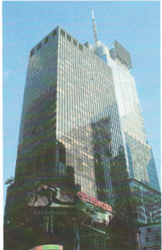
1500 Broadway in NYC is the site of a coil cleaning study.
