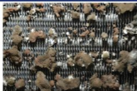
FIGURE 1 Tampa, Fla., downstream cooling coil surface fungal colonies before coil UVGI (left) and after 13 months of coil UVGI (right). 2
