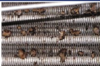
FIGURE 1 Tampa, Fla., downstream cooling coil surface fungal colonies before coil UVGI (left) and after 13 months of coil UVGI (right). 2
